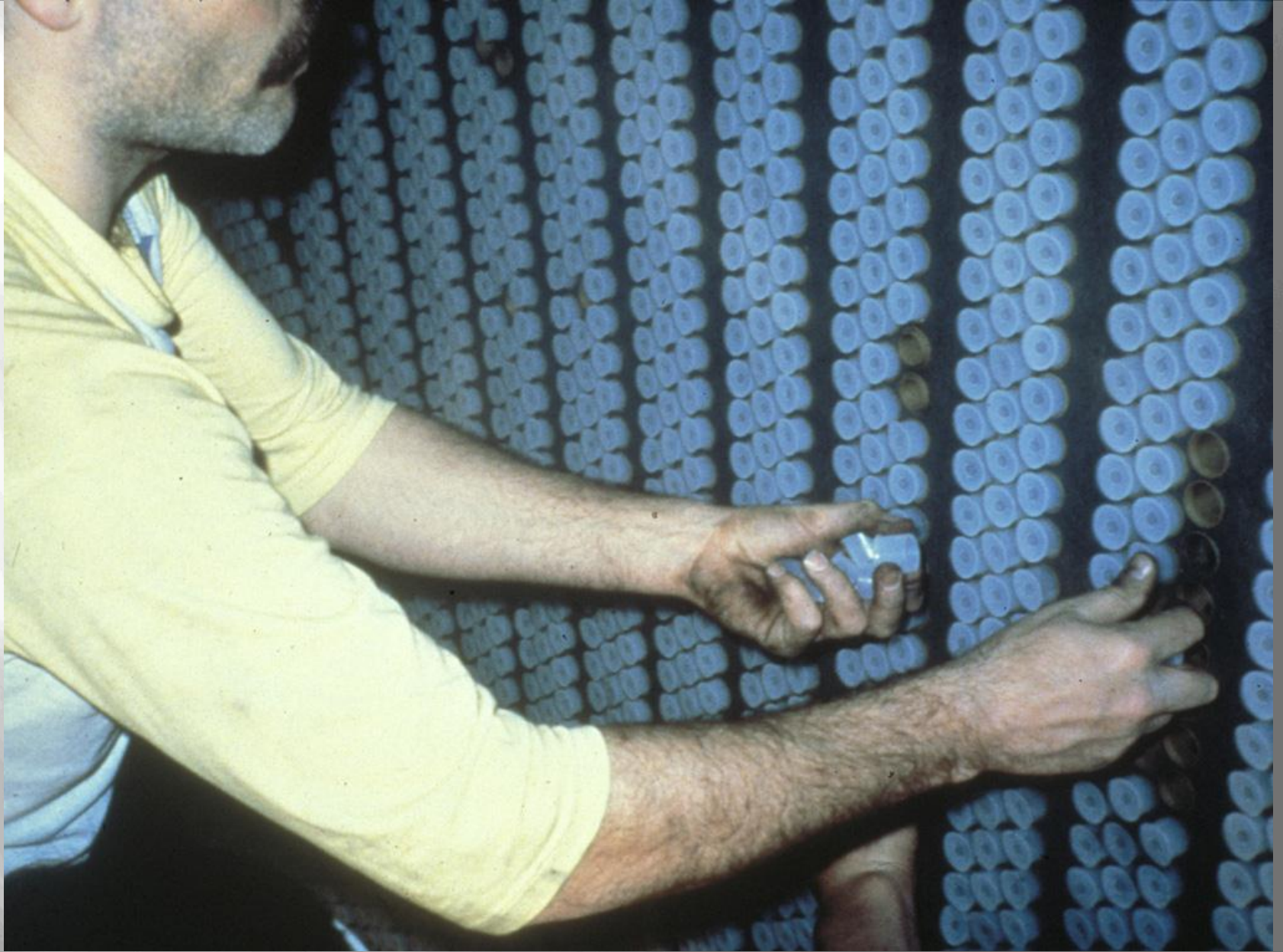
Coating plugs installed
